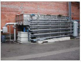
Floating is that operation through which solid substances, suspended or in emulsion, are separated from the liquid, either using their low specific weight either causing their floating through the injection of gas flow. In both cases we obtain the advantages of Archimede's principle for the bodies immersed in a fluid. This
